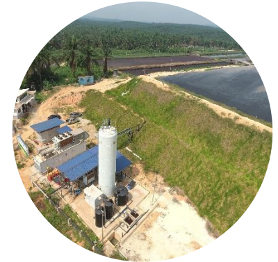
Methane Capture Plant at Kilang Sawira Makmur POM
