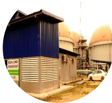
Methane Capture Plant at Endau POM
