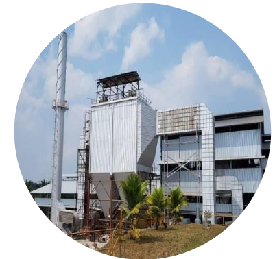
Double Field Electrostatic Precipitators (ESP) commissioned at Rompin POM
