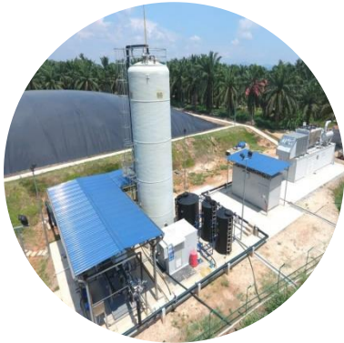
Methane Capture Plant at Cheekah Kemayan POM
