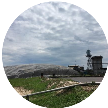
Methane Capture Plant at Prosper POM
