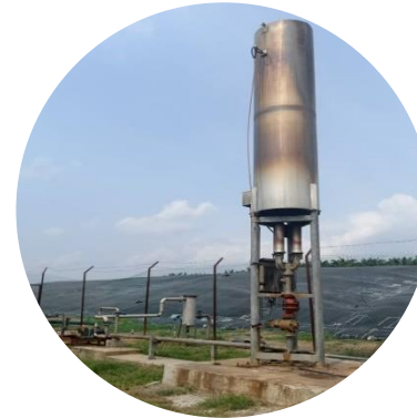
Methane Capture Plant at Kilang Kosfarm
